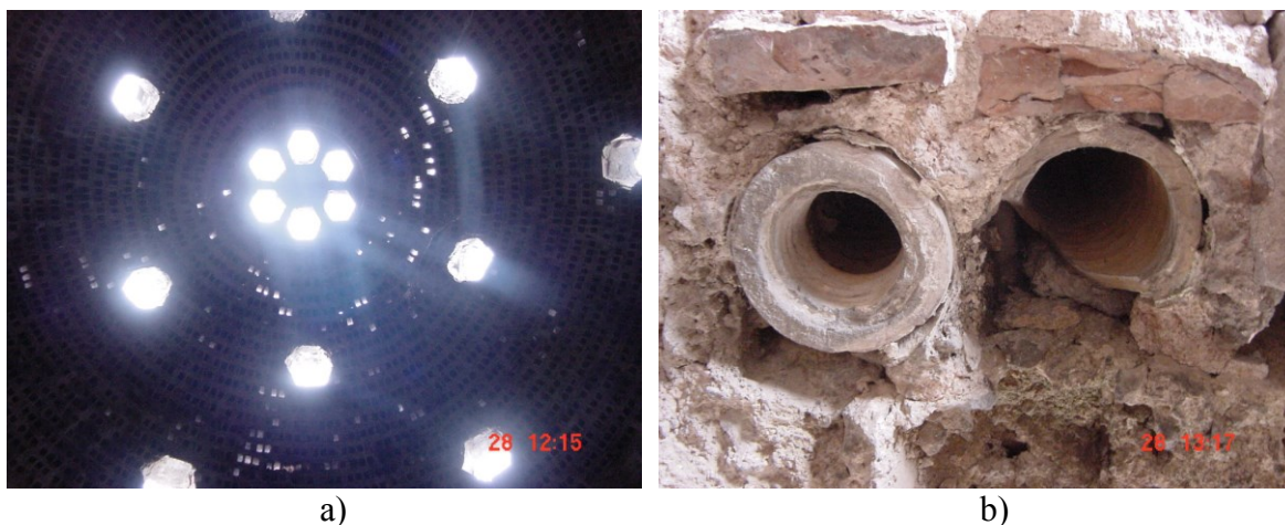
Fig. 8. Hammam in 2002: a) north-east dome; b) ceramic pipes
