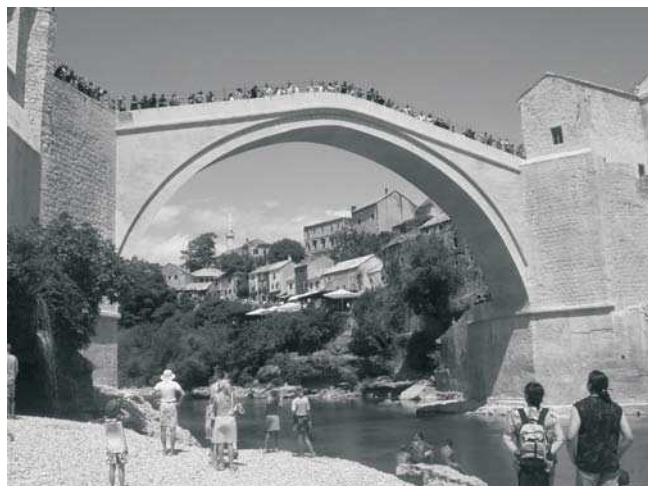
Fig. 29: New Old Bridge today
