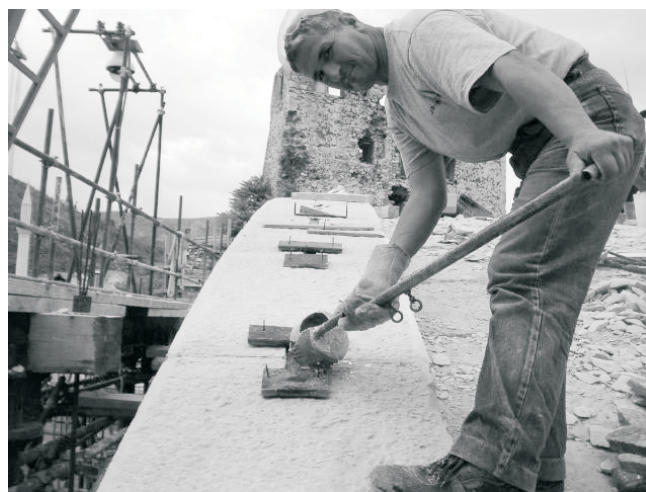
Fig. 24: Pouring the lead
