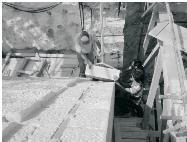
Fig. 16: Assembling the cornices
