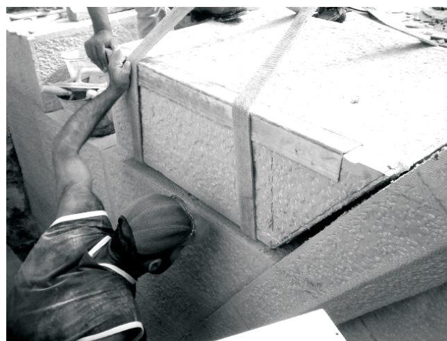
Fig. 18: Assembling the spandrel stones
