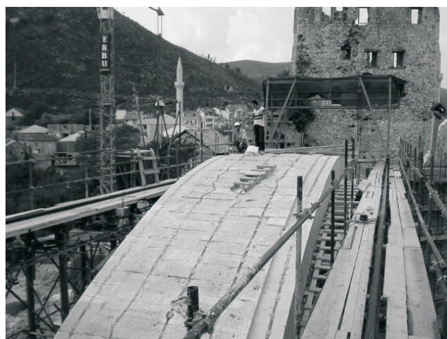
Fig. 12: Load bearing arch completed
