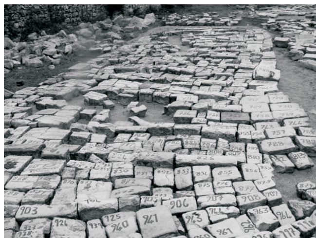
Fig. 8: Pavement stones in their new location
