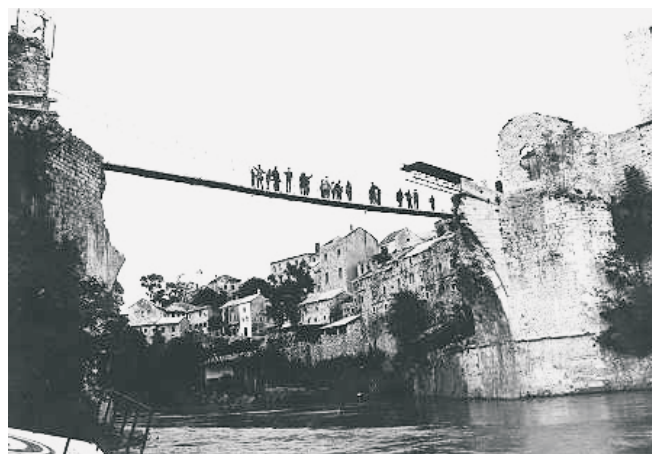
Fig. 3: Destroyed bridge – south elevation
