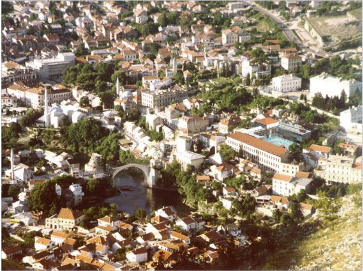
Photo-montage of the restored and converted complex in its existing surroundings
