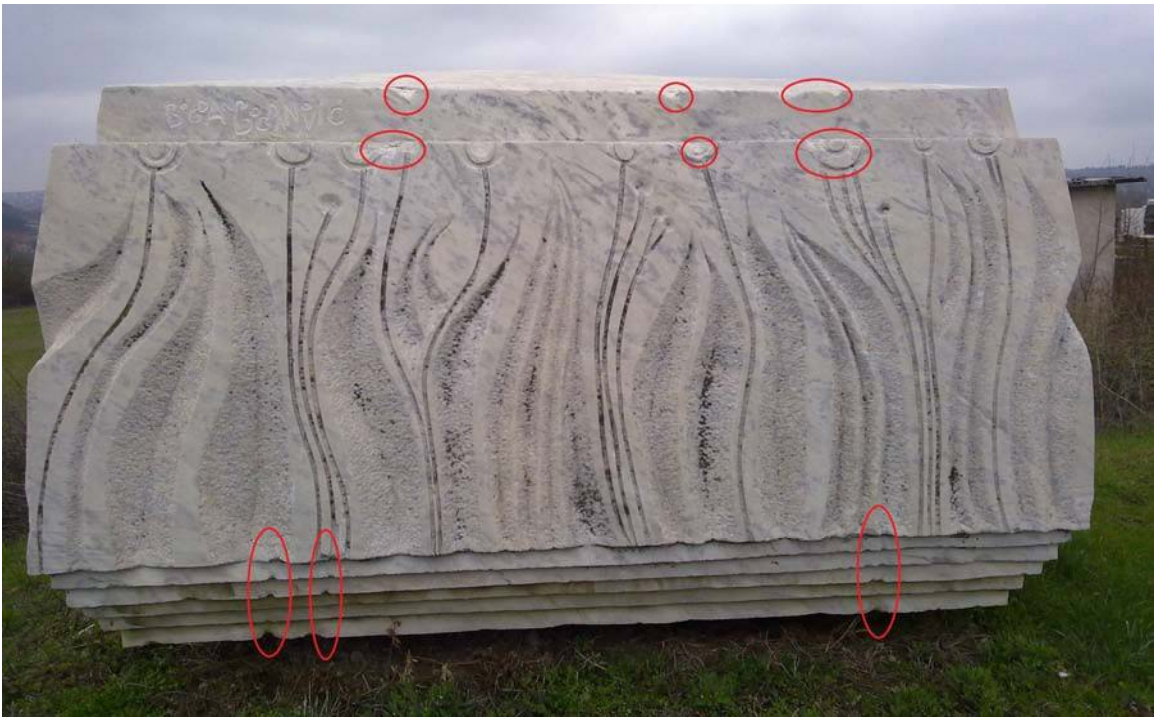
Fig 2.18.9 Detail highlighting concentrations of cracks and chips in the monument
