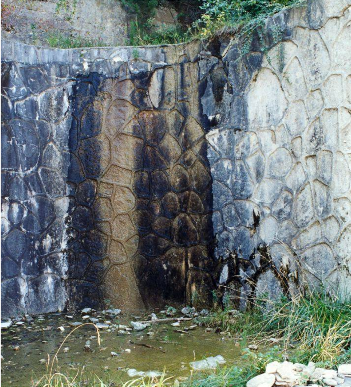
Fig 4.6.6: Water damage to alcove, 2000
