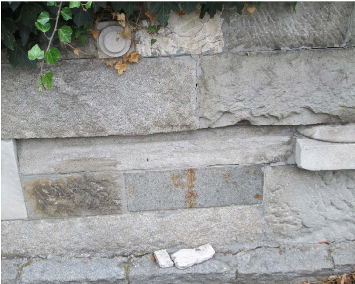
Fig 2.1.3 Bursting, cracking and erosion on the memorial pathway
