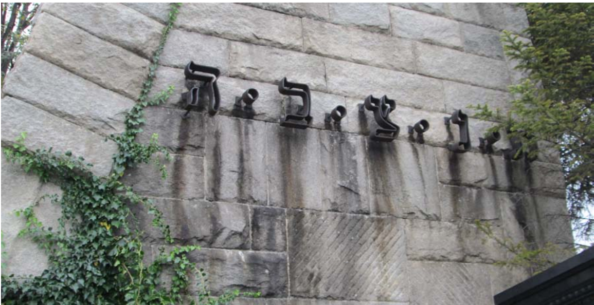
Fig 2.1.5 Staining from metal elements on the monument
