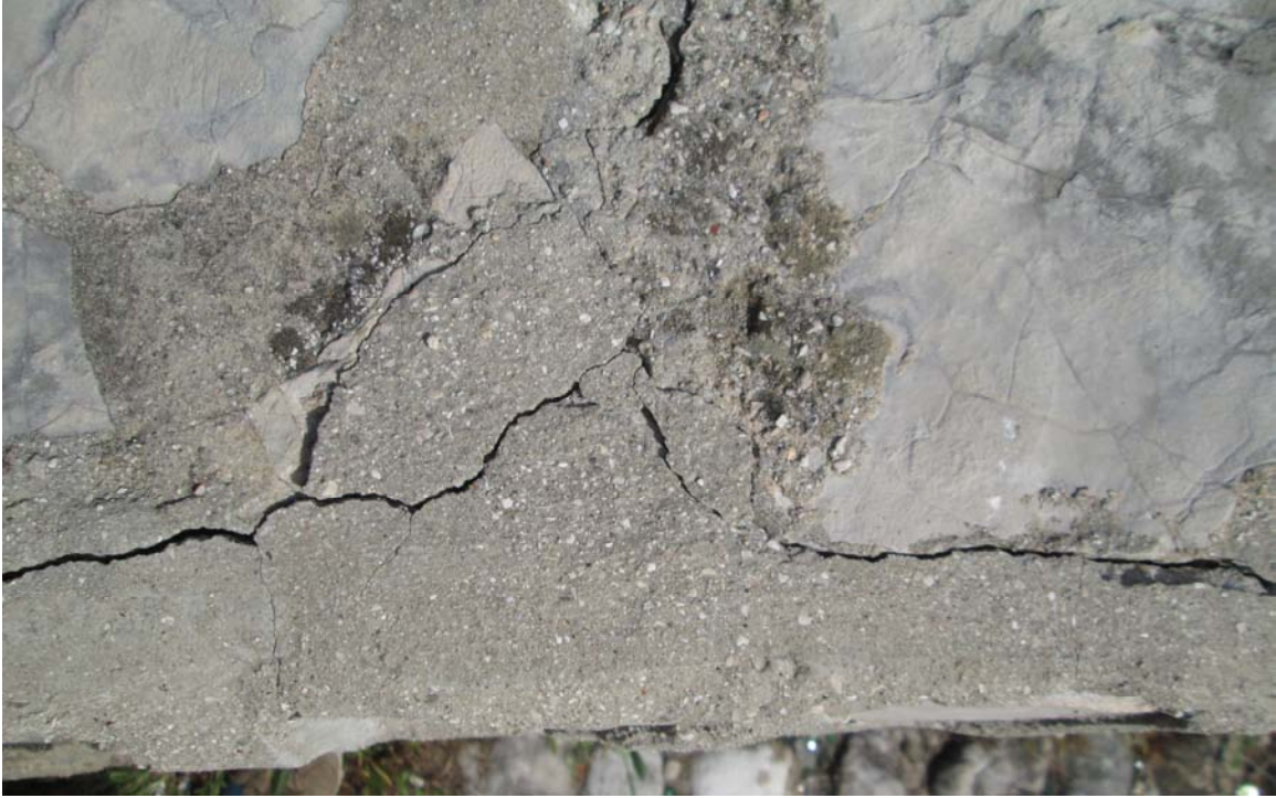
Fig 6.18: Cracks in repaired mortar, April 2013
