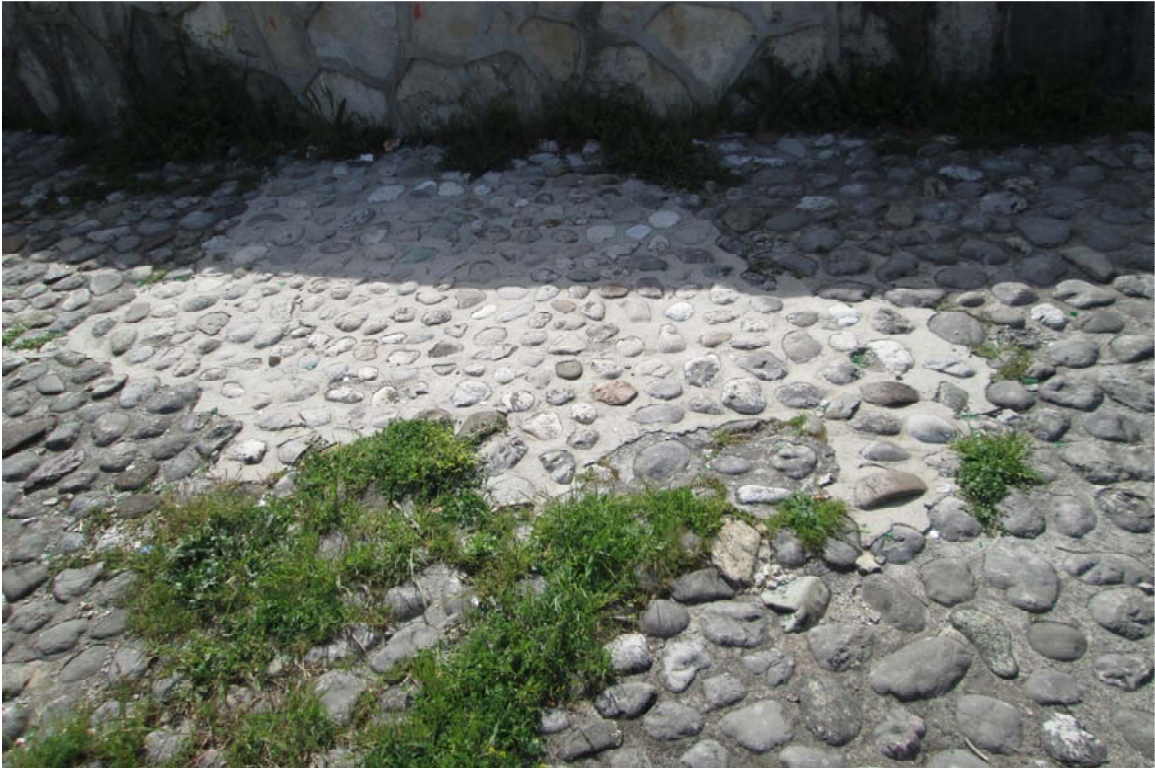
Fig 6.19: Replaced cobbles with deteriorating mortar, April 2013
