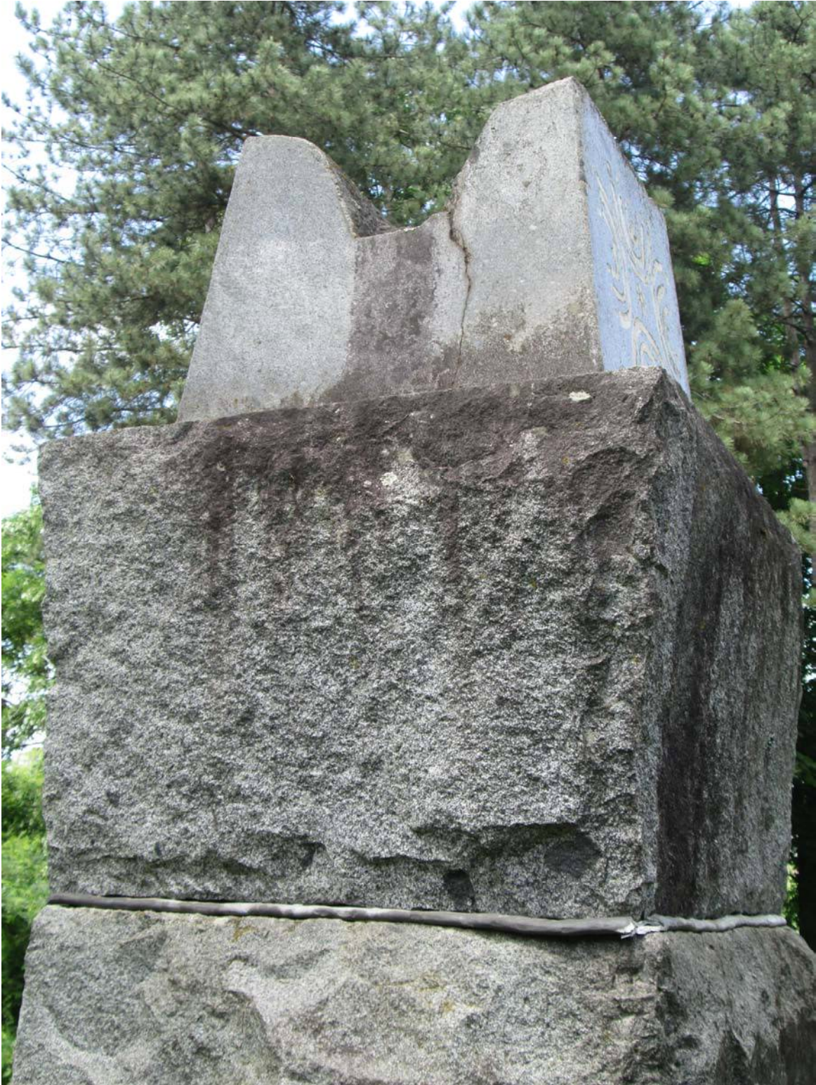
Fig 2.8.9 Cracks in the šajkač on top of one column
