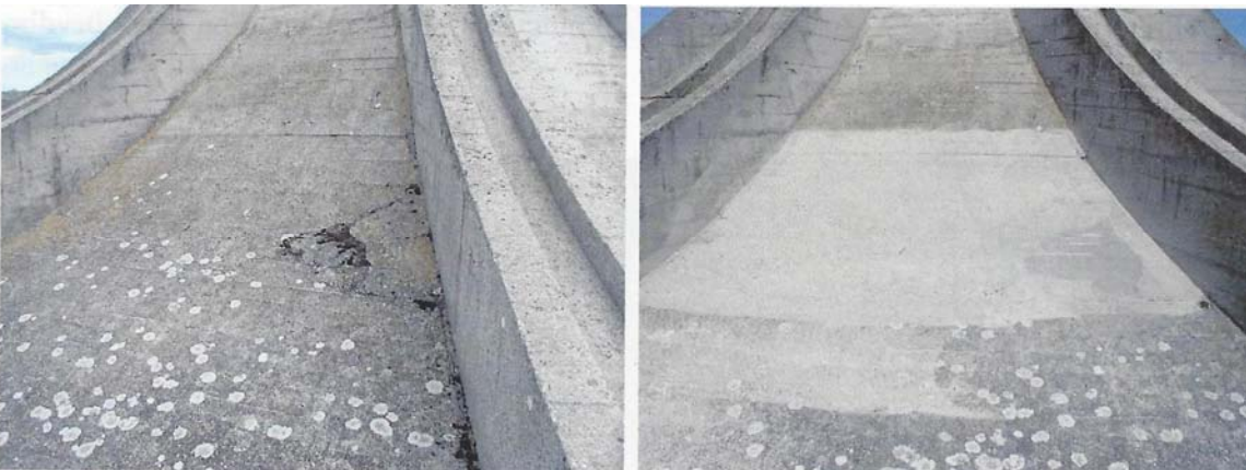
Fig 2.6.8: Treatment of biological growth and wartime damage
