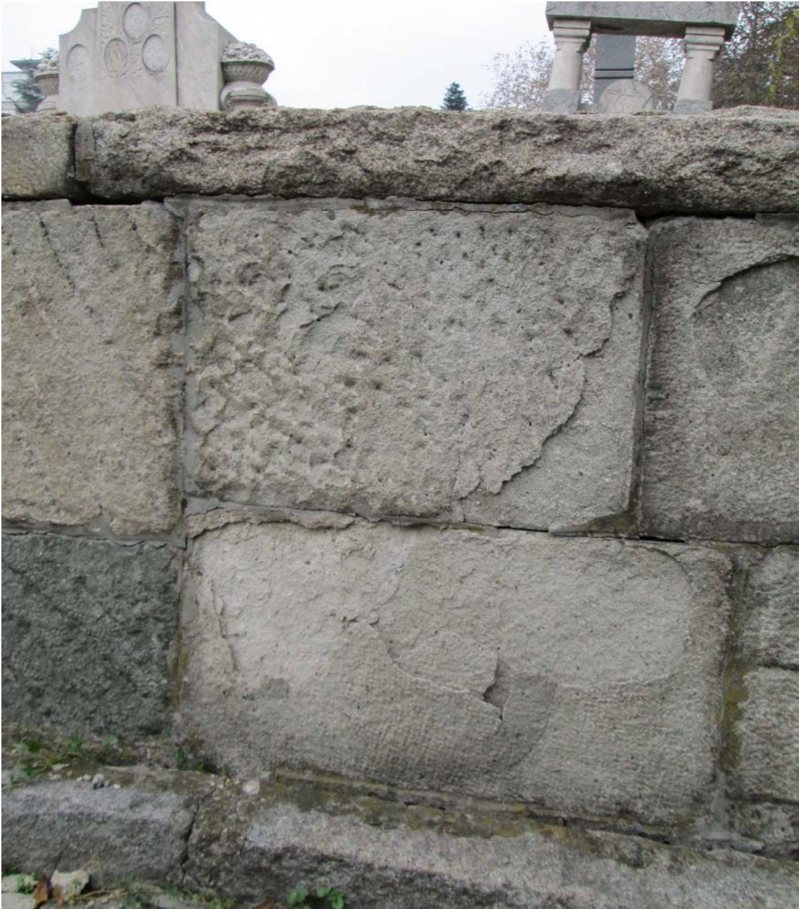
Fig 2.1.7 Delamination on the memorial pathway
