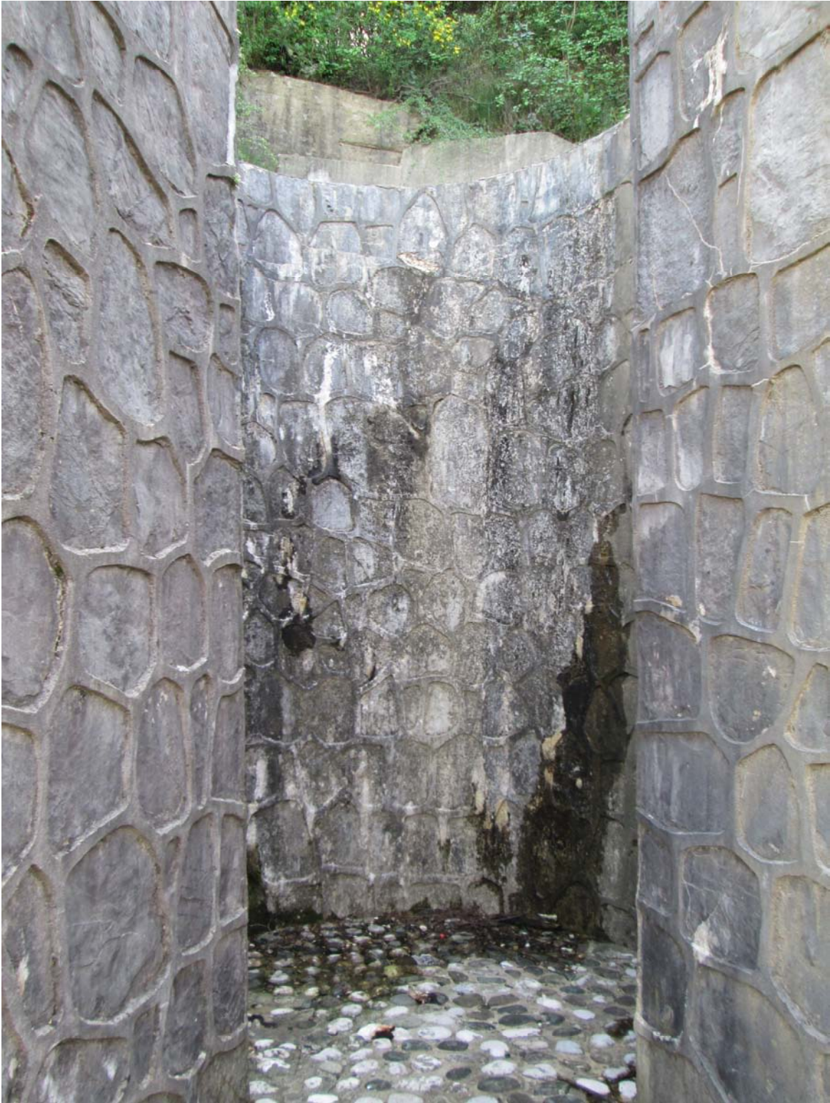
Fig 2.5.30 Current problems due to drainage failure, 2013
