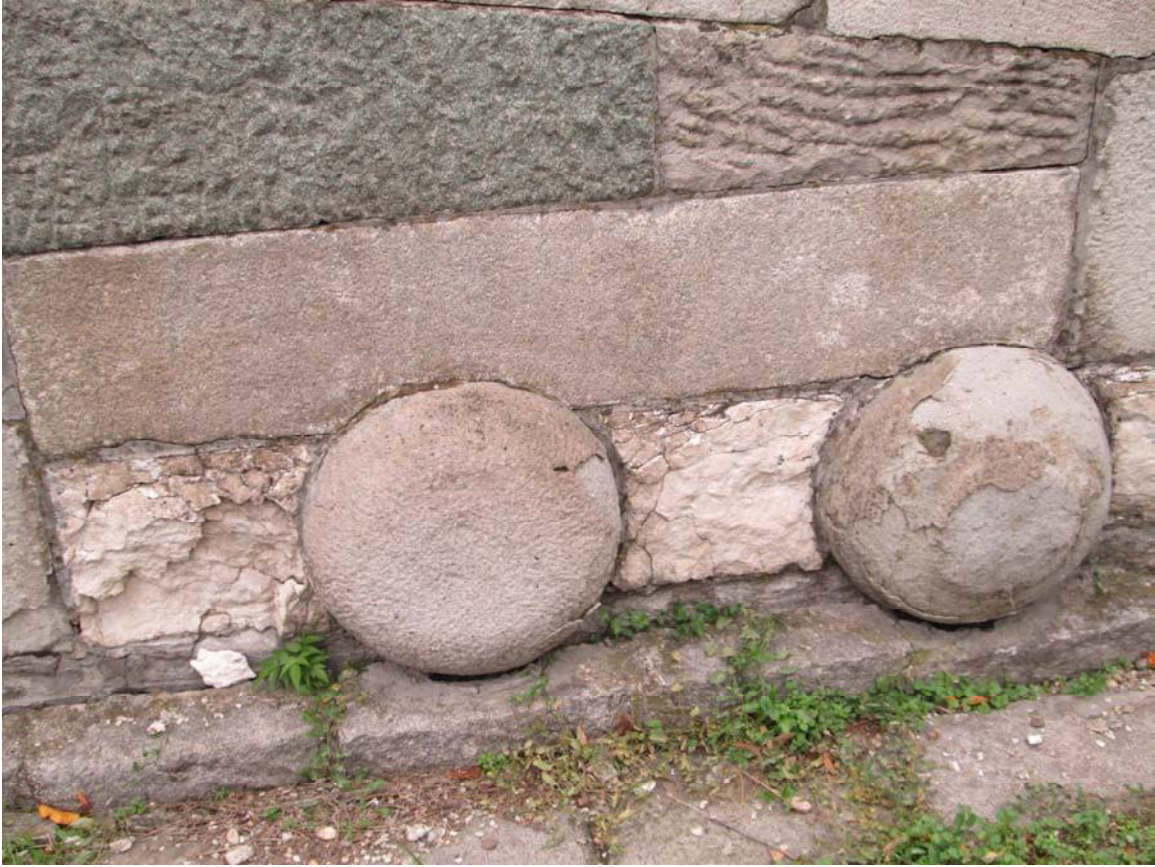
Fig 2.1.4 Delamination and bursting on the memorial pathway
