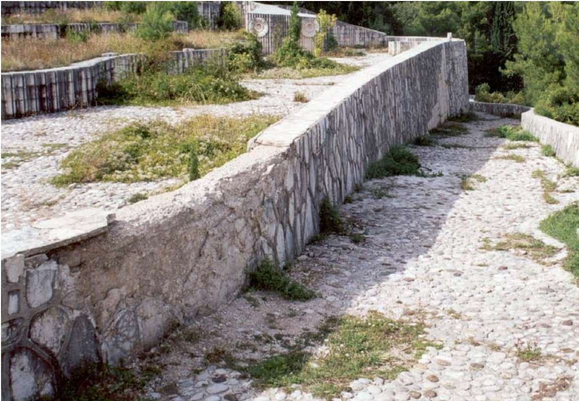
Fig 4.6.5: Wall cladding missing due to shell impact
