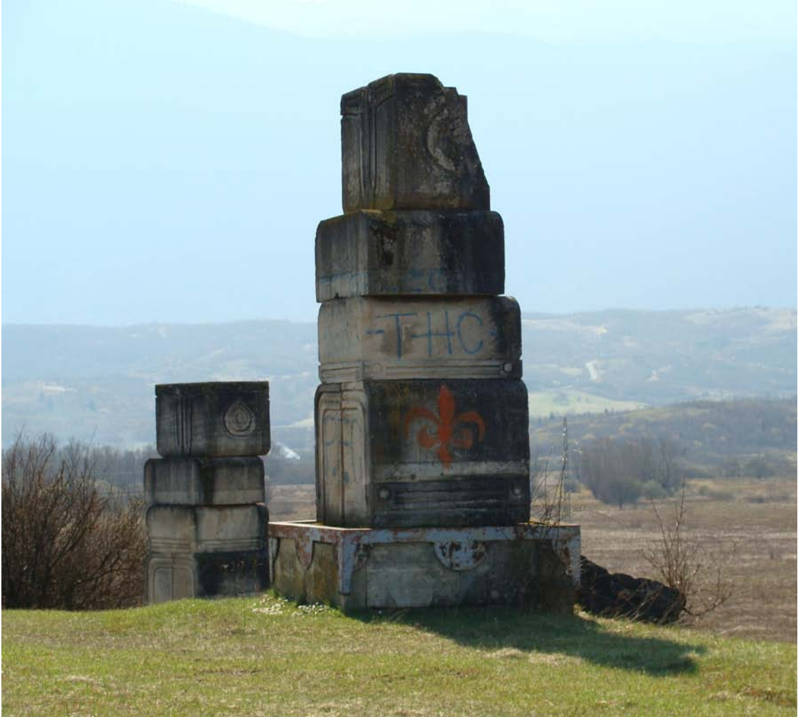
Fig 2.19.12 Column with uppermost portion badly damaged by shell impact
