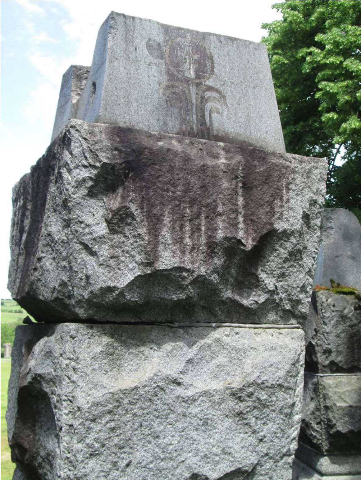
Fig 2.8.10 Heavy staining to the uppermost portion of a column
