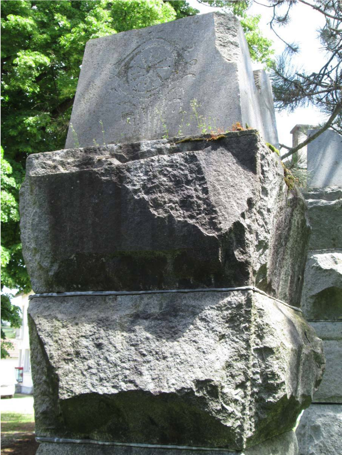
Fig 2.8.8 Damage to upper portions of one of the columns
