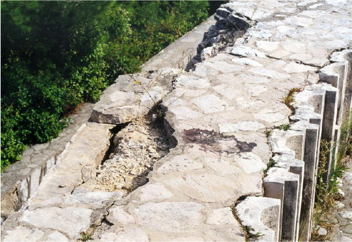
Fig 4.6.4: Cracks in the walls, 2000
