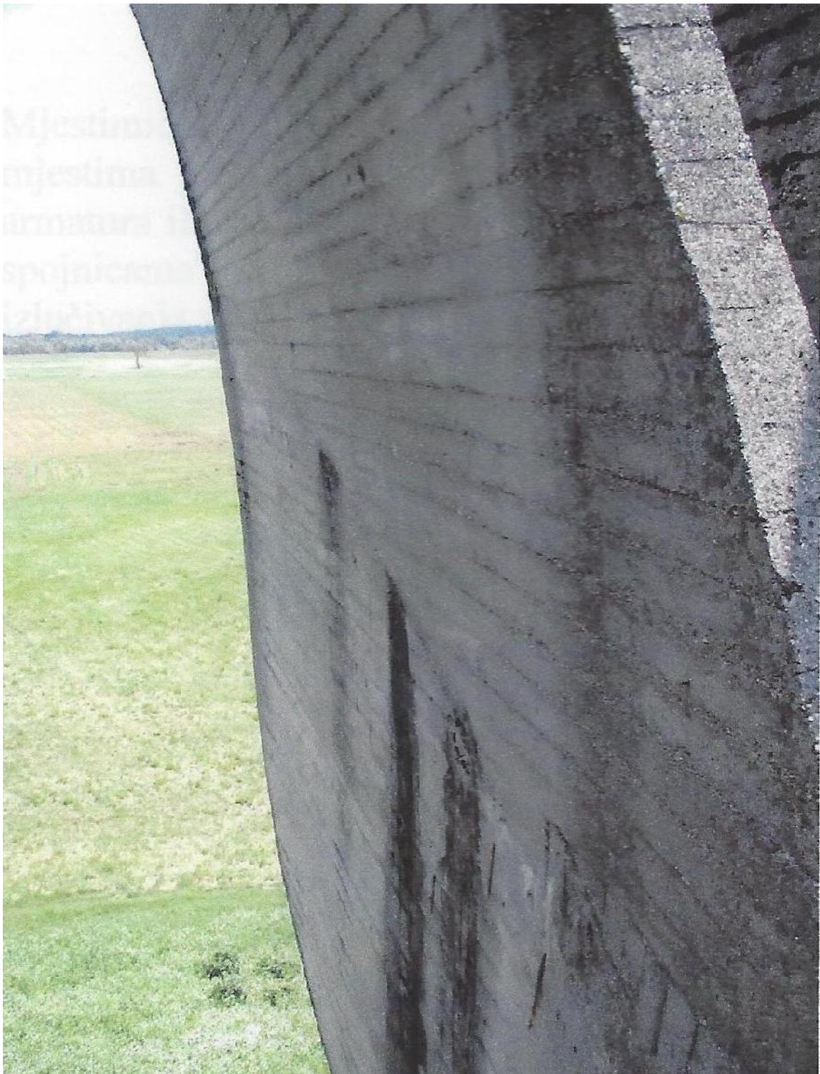
Fig 2.6.5: Staining from corrosion penetrating the monument
