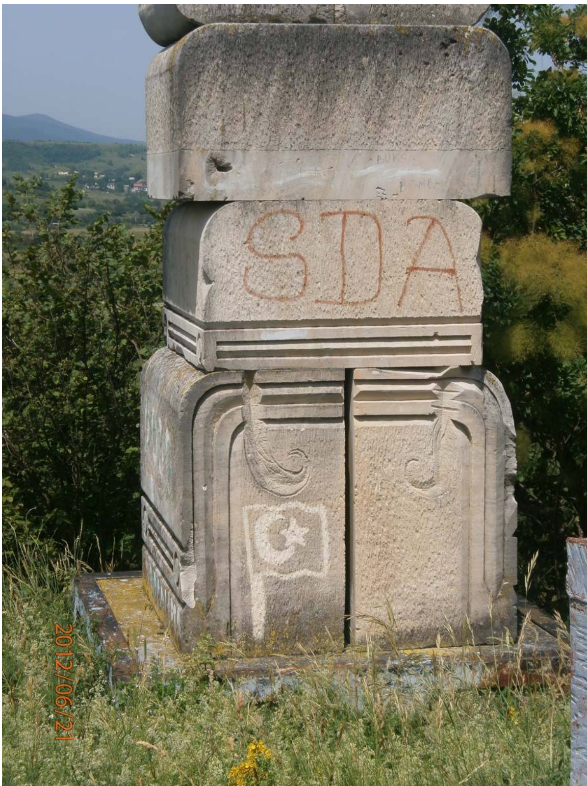
Fig 2.19.11 Column bearing evidence of a bullet hole (upper left), graffiti using ink (centre) and an unknown corrosive material (lower)
