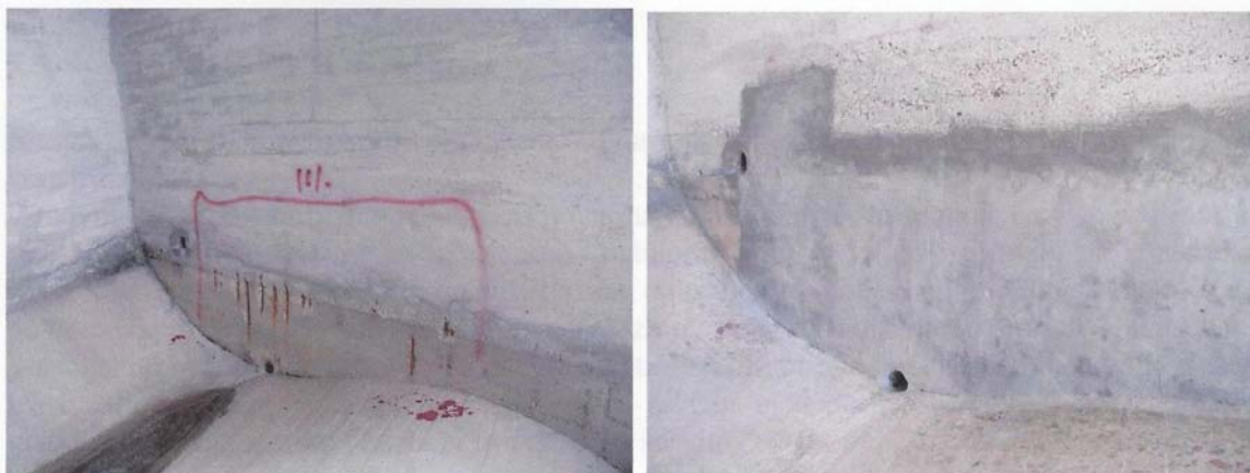
Fig 2.6.4: Restoration of corroded steel, before and after
