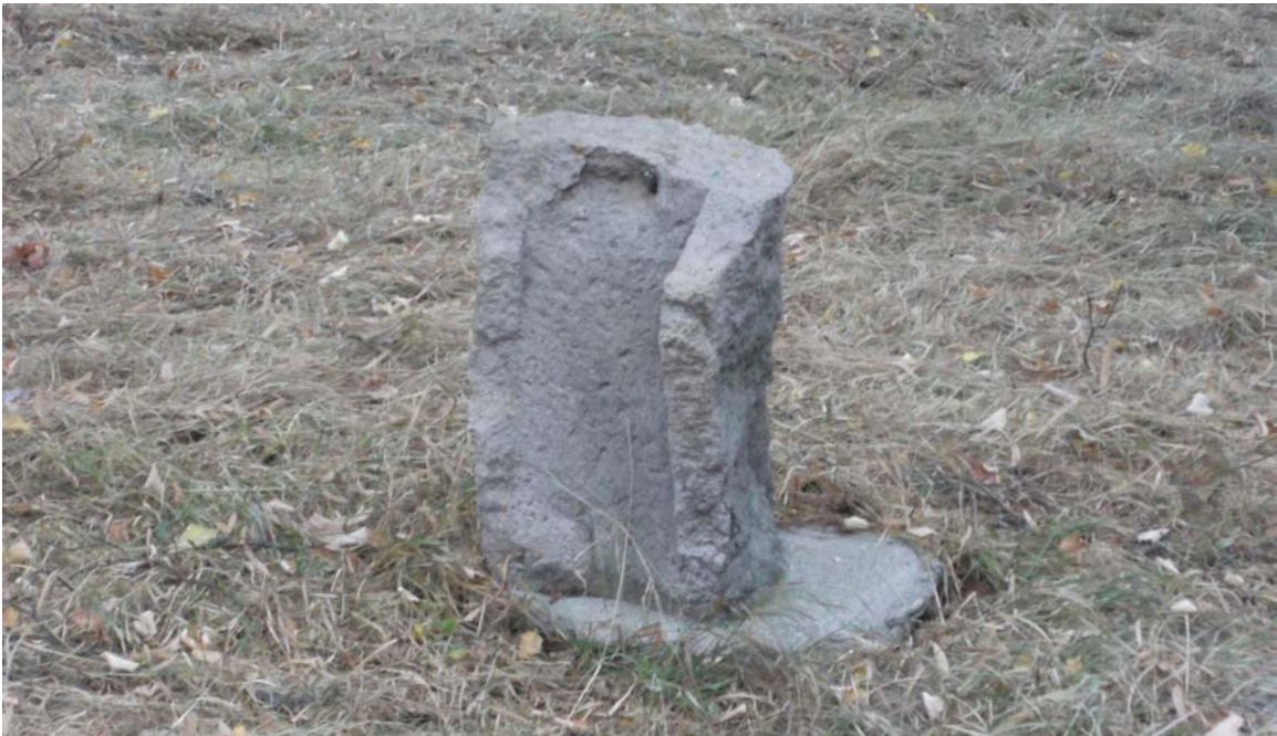
Fig 2.7.8 Damaged lantern fitting
