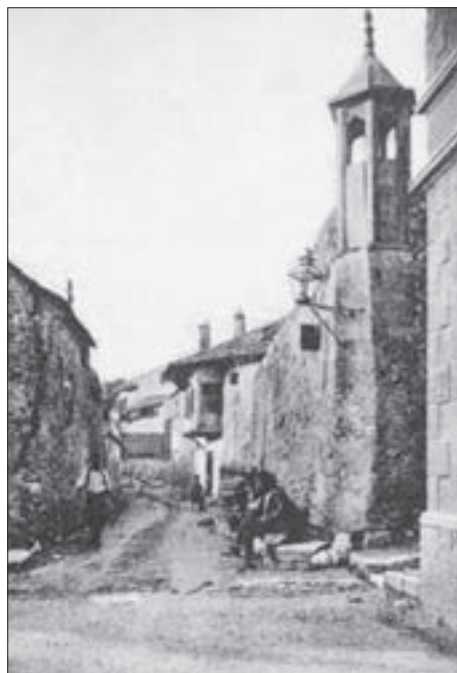
SL. 13. TIPIČAN SOKAK FIG. 13 A TYPICAL STREET
