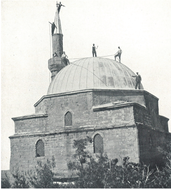
Plate 5: Hersekzâde Ahmed Paşa Câmii During ca. 1935 Restoration
